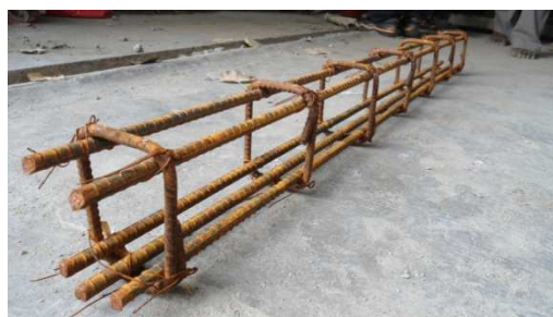
Figure 4: Reinforcement of Beam
